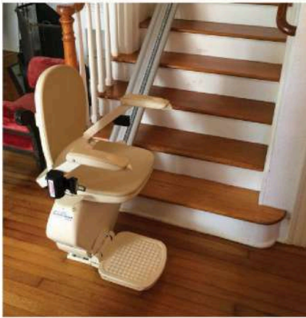
(A-4) STAIRCASE ELEVATOR
